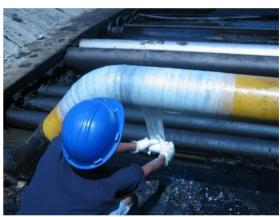
Unique Polymer Systems have developed a special braided GLASS FIBRE TAPE that, when used in conjunction with the UPS Standard Resin and Hardener, offers the ultimate in both LEAK SEALING and PIPE PROTECTION
